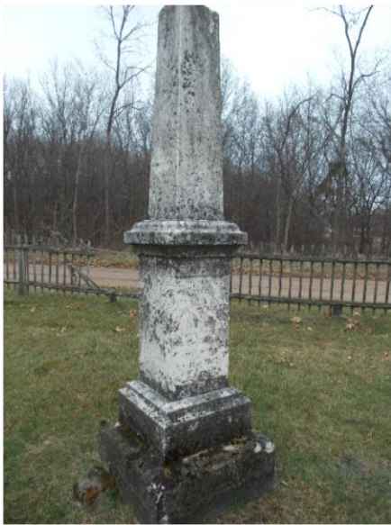
Civil War Monument in need of cleaning and repair
