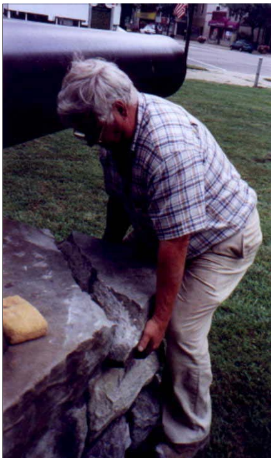
Ron Aves removes the corner for repair.
